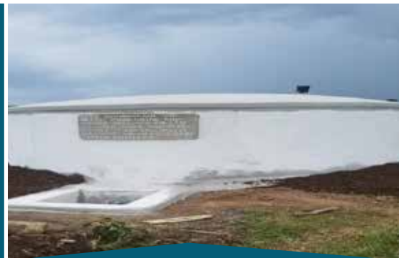
TPC PLC continues to partner and work with institutions that assist with water issues in various villages. This year, Twiga Cement is working with an NGO under the Catholic Diocese of Singida, that is helping the community to build water tanks in Sakaa and Misughaa villages, in singida region "Water Tank Project - Singida"
